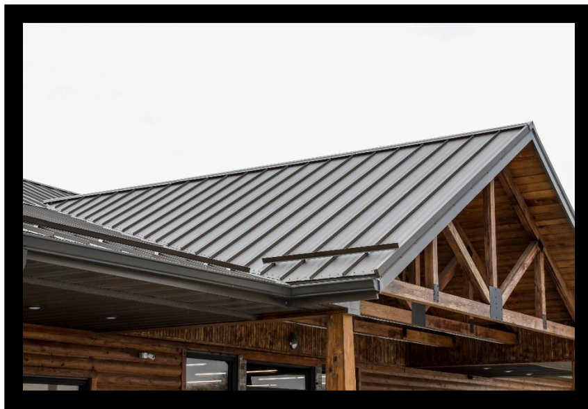
Standing Seam Roof
